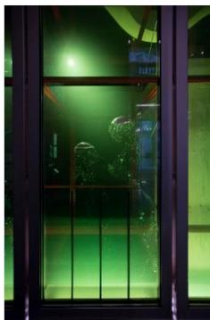
The exhibition includes a series of full-scale SolarLeaf© Algae Façade prototype panels, as an example of how Arup continues to innovate the field of building design today. SolarLeaf© is a new experimental bio-reactive building façade system developed by Arup with Colt International. It uses microalgae to generate renewable energy to heat buildings as an alternative and environmentally-friendly energy source.
