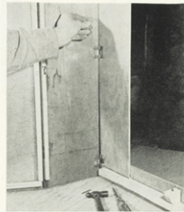
For easy disassembly, wings and proscenium are joined with loose-pin hinges, held with flat-head bolts (countersunk in the wood) and nuts.
